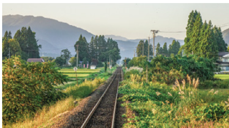
A railway in Akita
